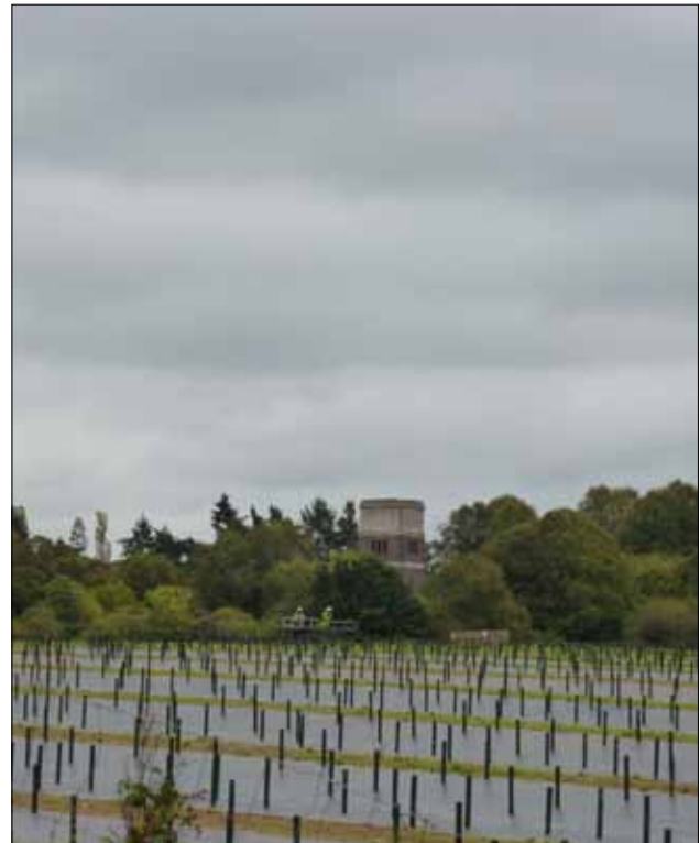
THE WATER TOWER IS VISIBLE FROM STATION FOOTPATH, WHILST THE REST OF THE SITE IS SCREENED BY TREES
