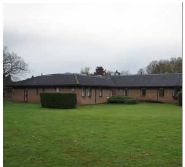
MILFORD HOSPITAL - 1980S OPERATIONAL BUILDING
