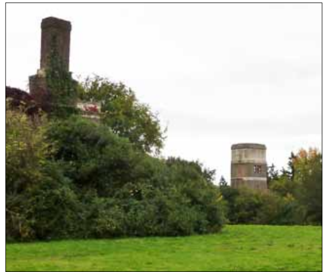
THE SITE IS CHARACTERISED BY A COMBINATION OF MATURE LANDSCAPE AND REDUNDANT BUILDINGS
